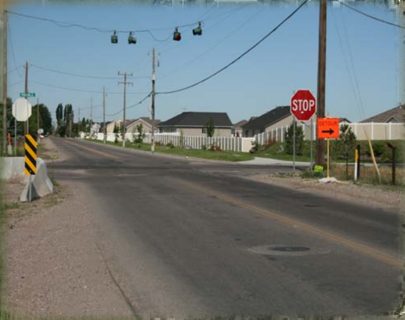
The intersection of Chubbuck and Philbin is identified as requiring intersection improvements such as a signal or roundabout.
